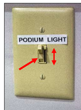
Podium Light Switch (on/off & dimming slider)
